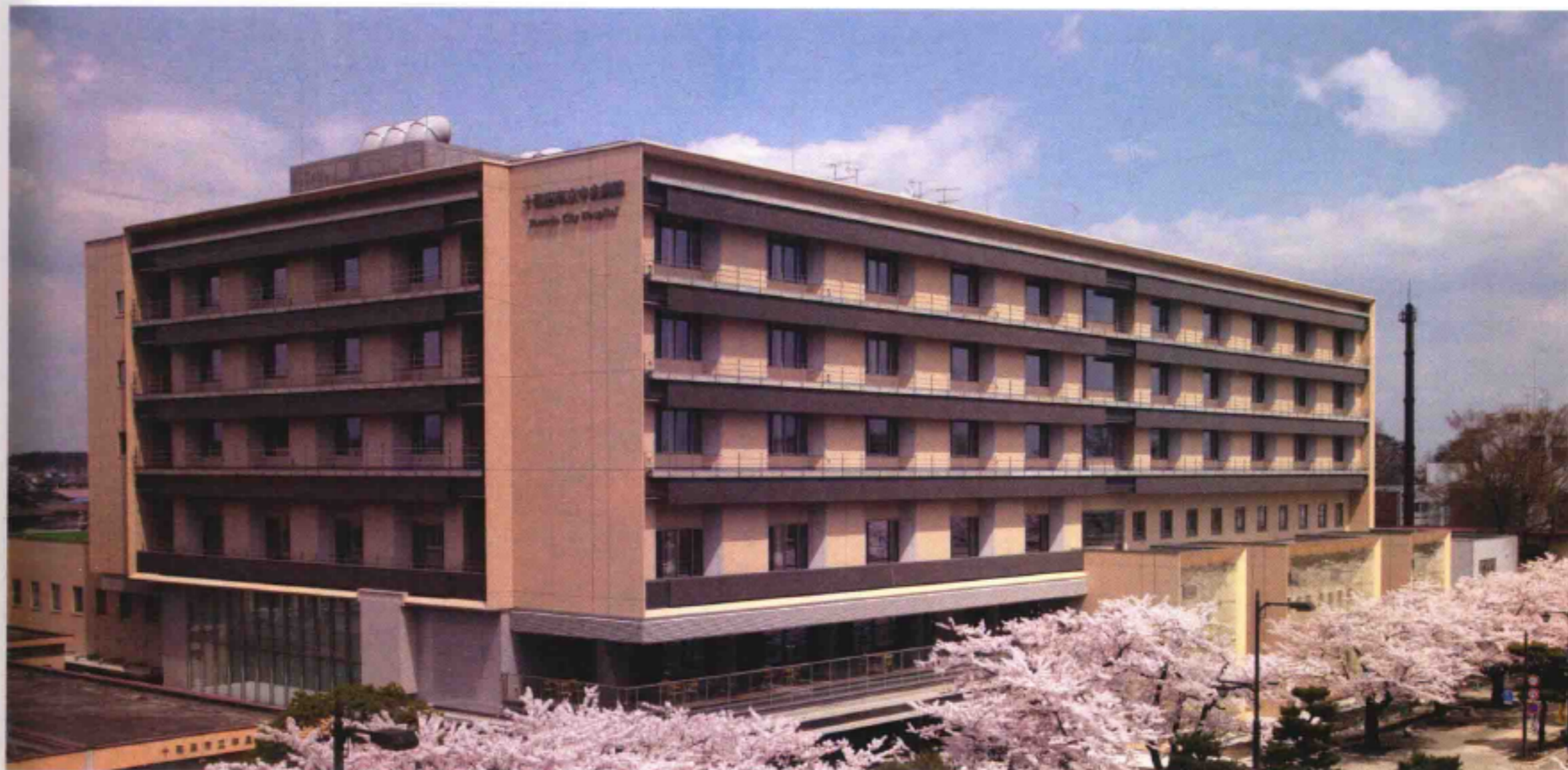
建筑外观与其所在的政府机关区建筑相称 Externals considered in accordance with the streets at the government office quarter
