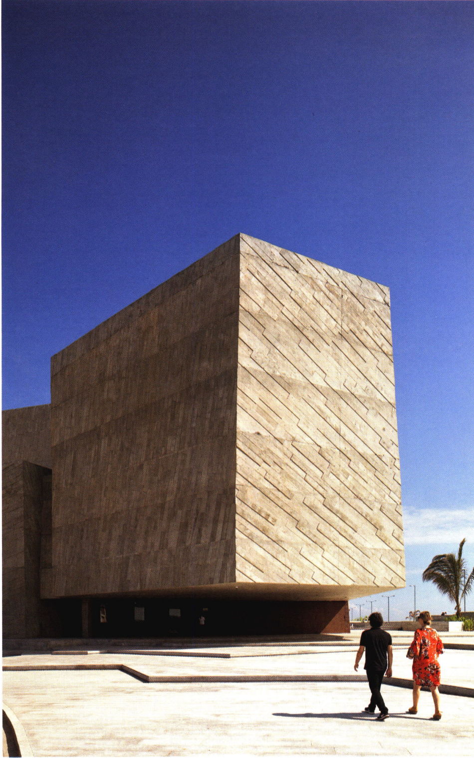
2 外景/Exterior view
