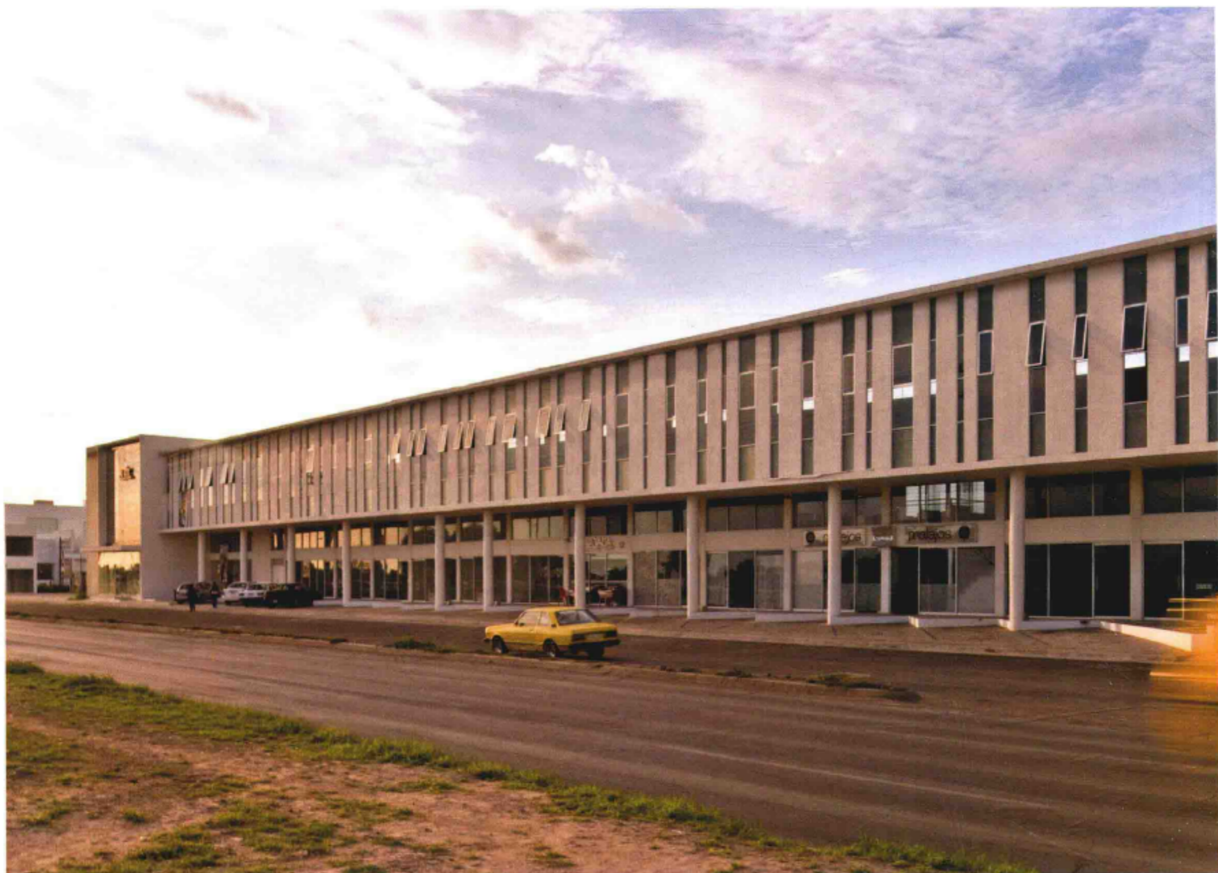
It is an almost 100-metre-long building, with a series of vertical strips used for ventilation by tip-up windows 建筑总长度近100米，竖条结构的窗户保证了通风
