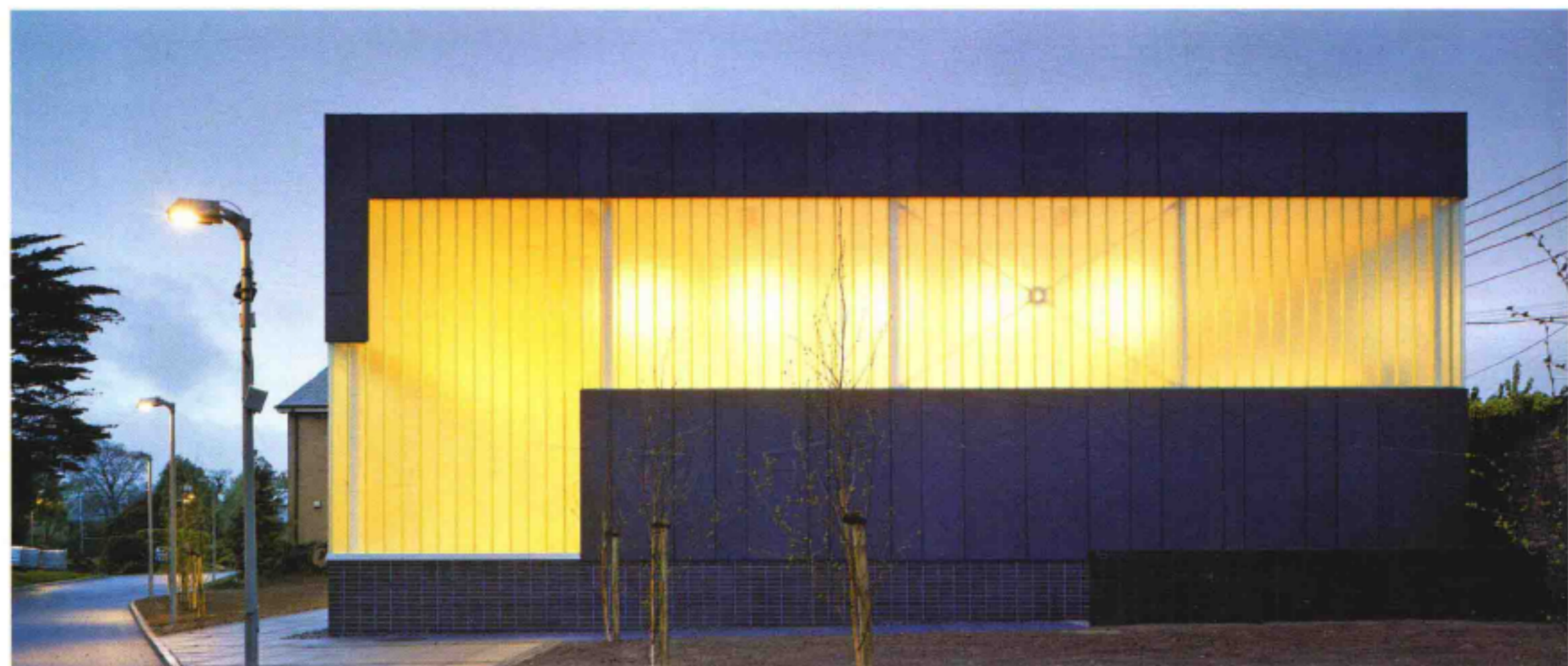
Front elevation's night view 建筑正面夜景
