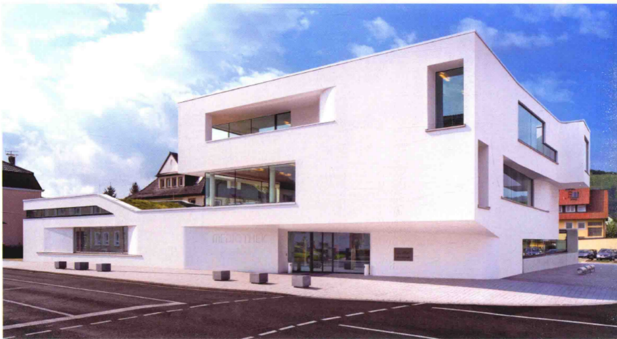
Main entrance in the daytime 主入口日间景色
