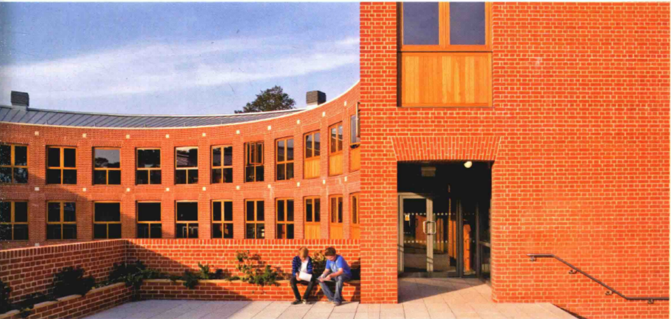
建筑外观 External view
