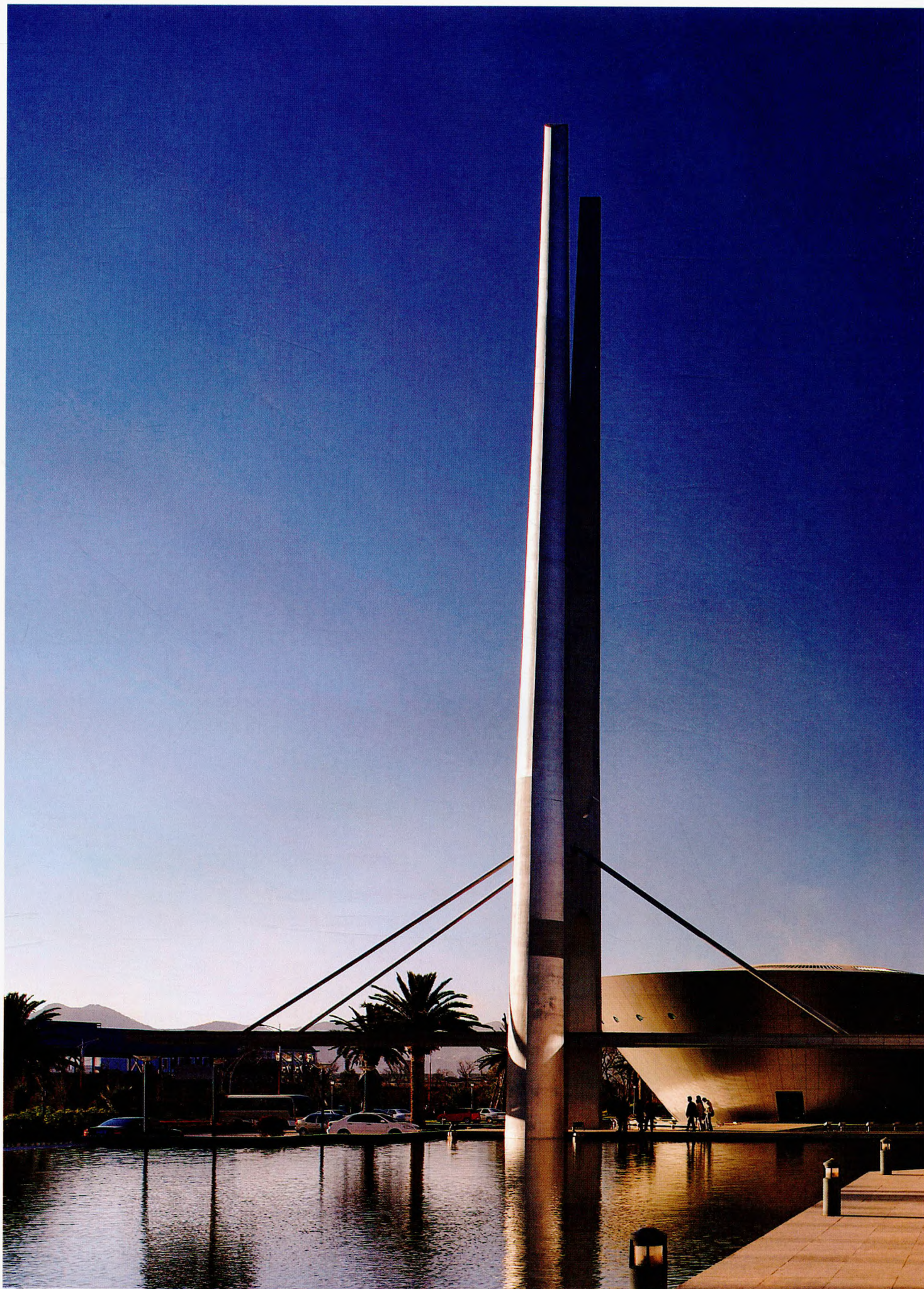
14 外景/Exterior view
