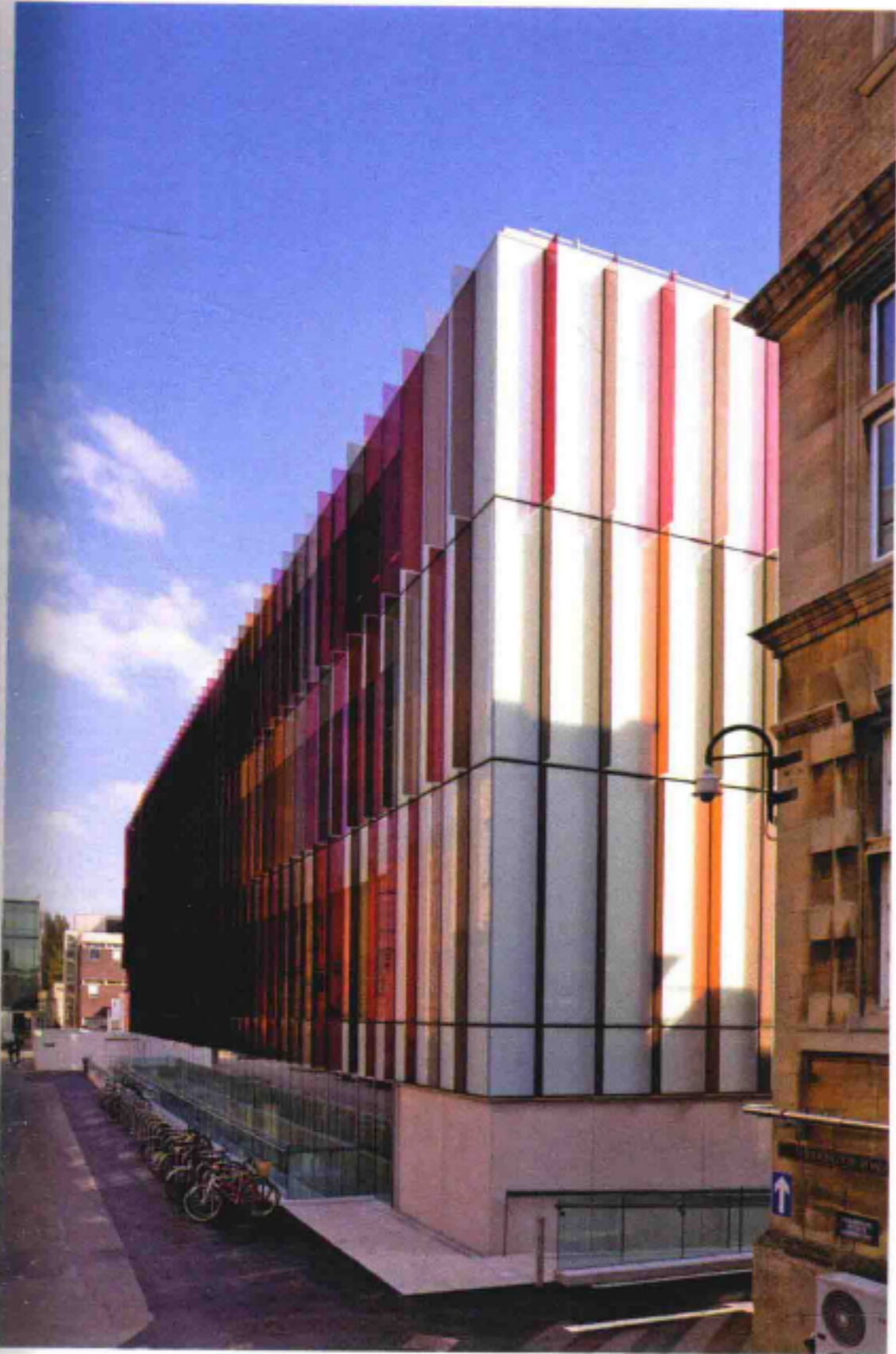
Coloured glass fins fixed vertically within the mullions wrap the full perimeter of the building 垂直于窗框安装的彩色玻璃片装饰着建筑的外围
