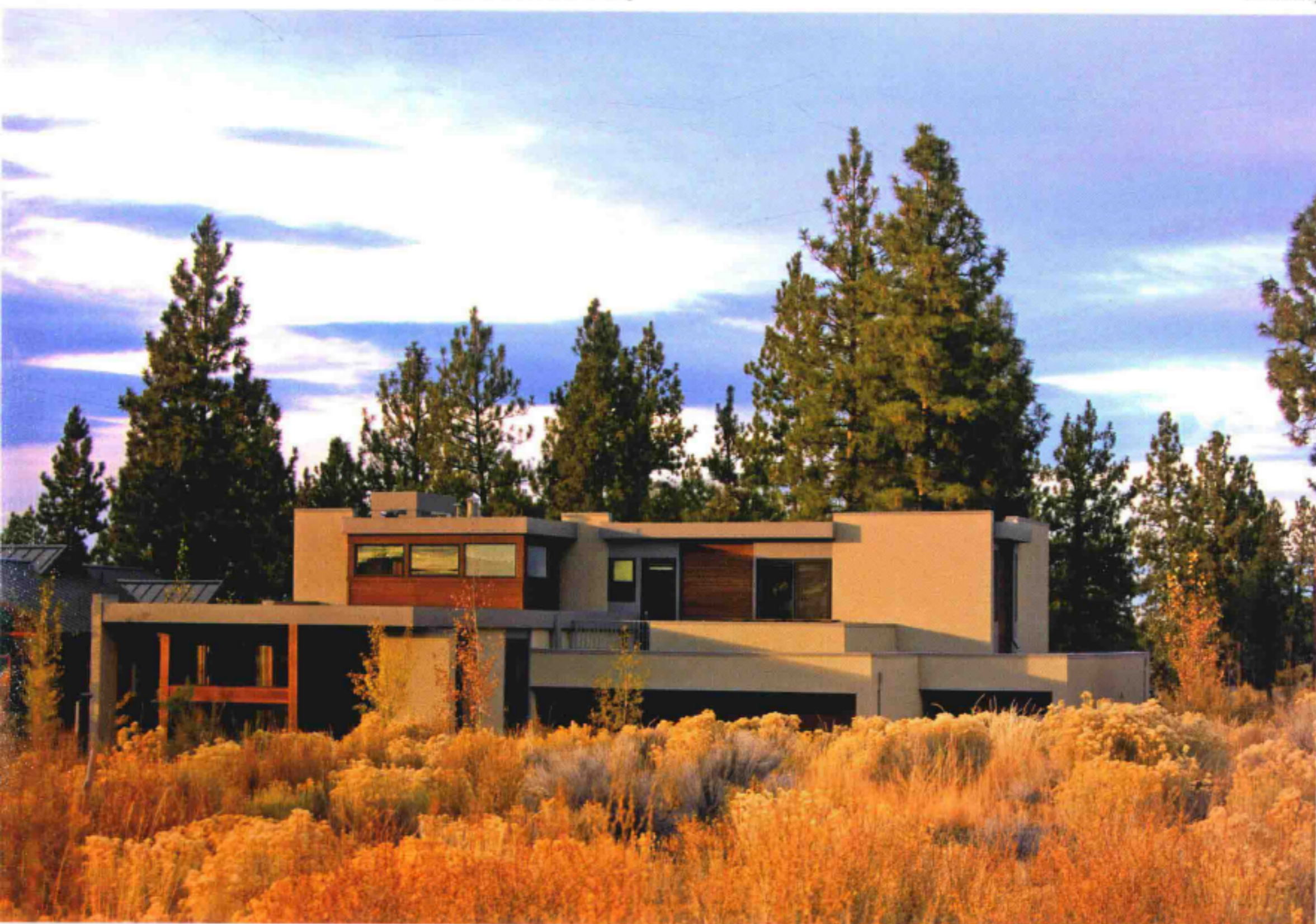
傍晚，建筑正立面 Front side in the evening
