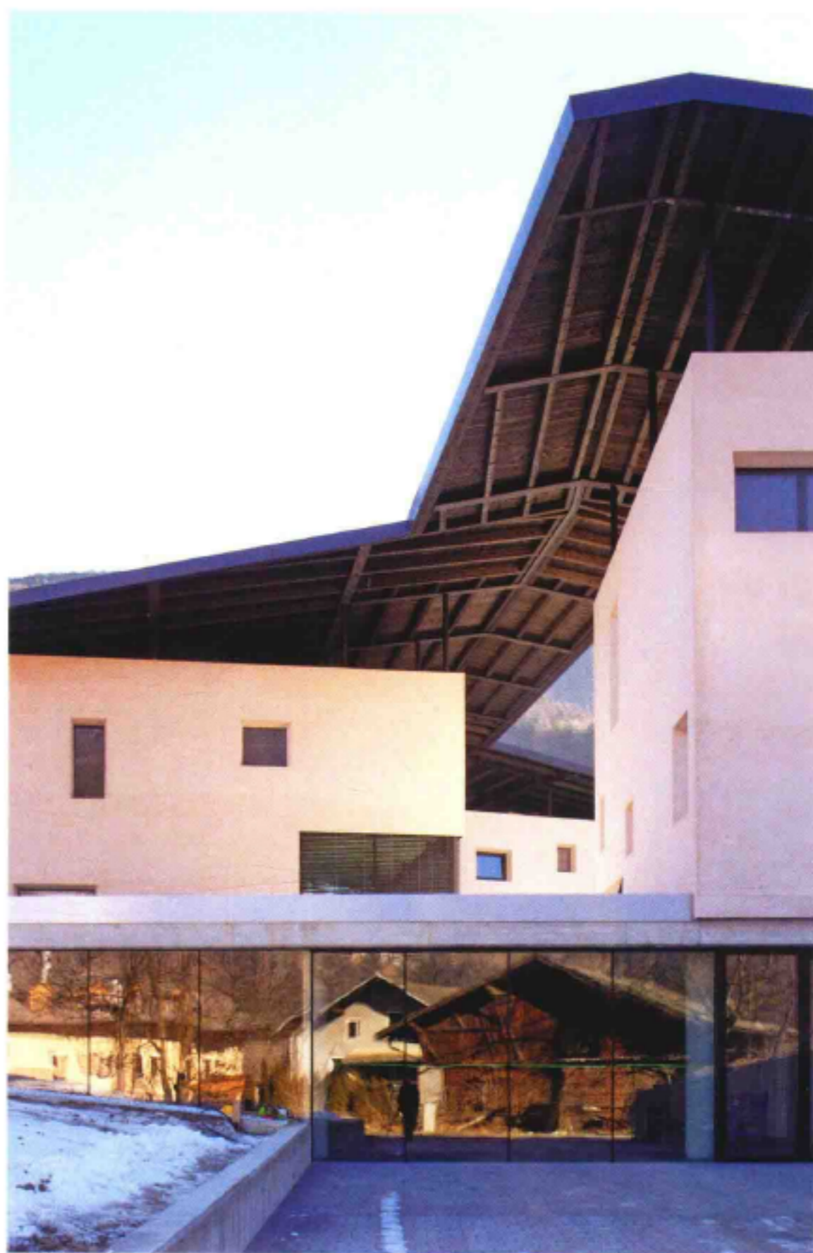
建筑侧面 Side view of the exterior
