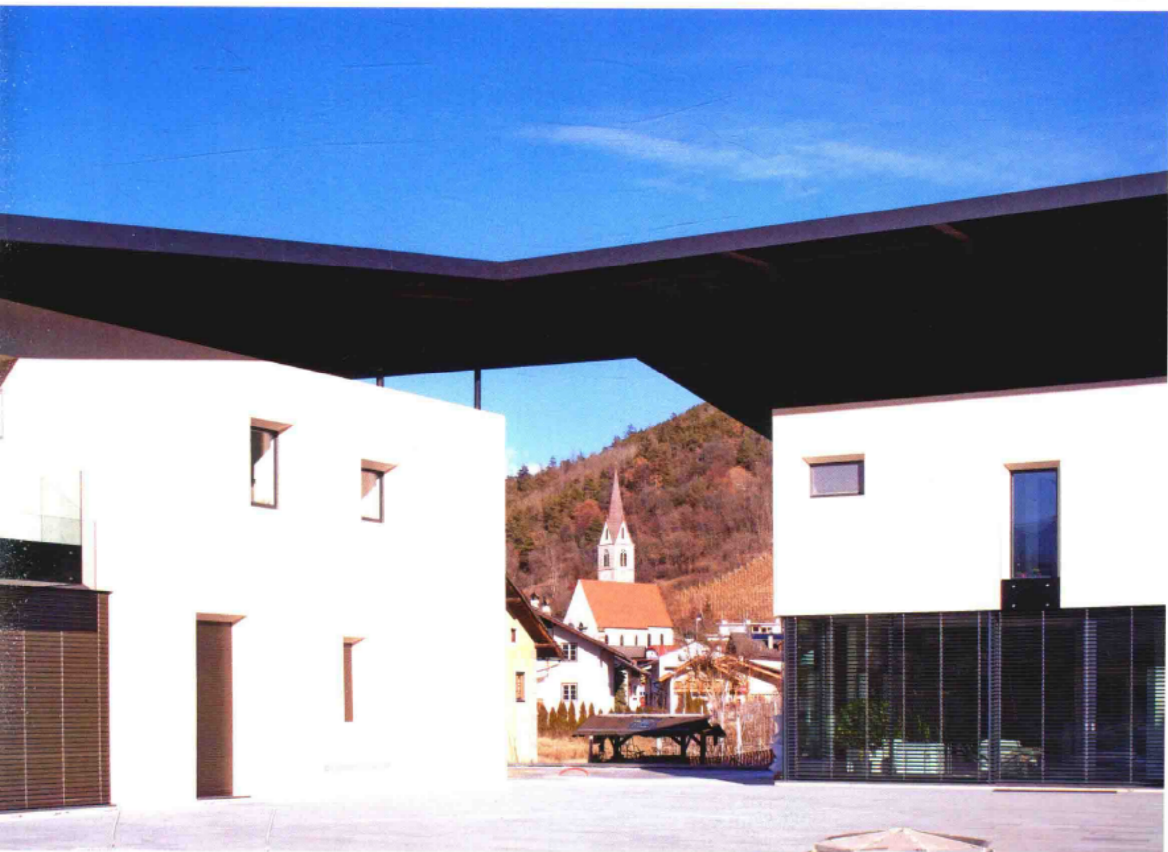
屋顶连接处 Rooftop connection
