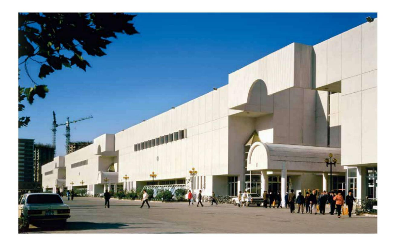
Hall No.2 to Hall No.5 are the first phase of the construction of the China International Exhibition Center. The four exhibition halls are connected by 3 connecting spaces. Considering the requirement of flexibility, each exhibition hall is defined as a 63mX63m square space. Inside the exhibition hall, a gallery corridor is pulled out of the enclosing walls at 4.5m height, which not only extended the space for exhibitions, but also diversified the spaces from both interior and exterior.
